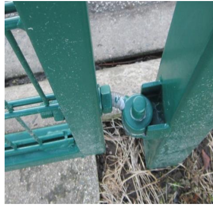
Photo 2: Bent stem of eye bolt ( at same school)
