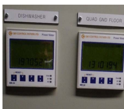
Sub-meters showing where the energy is used
